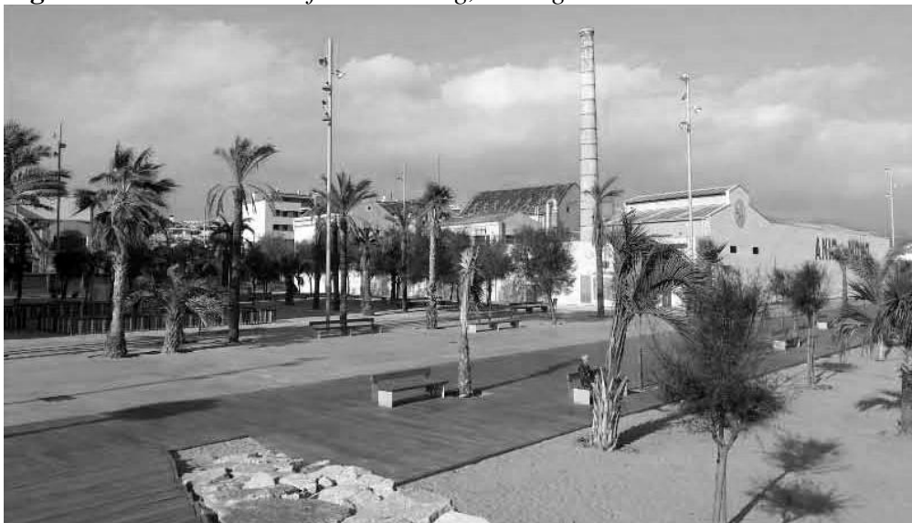
Figure 7. The West Side of the Building, Facing the Sea
