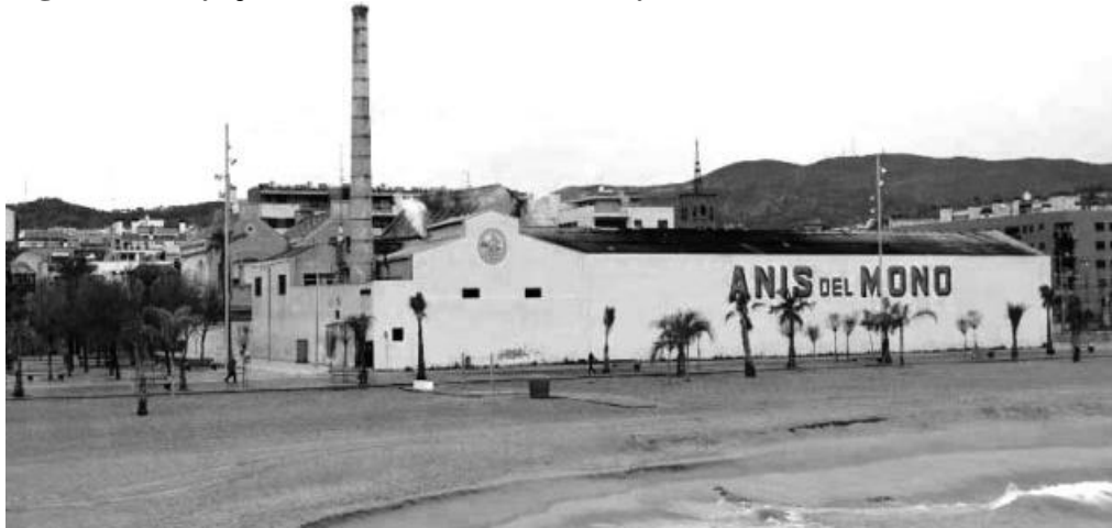
Figure 4. Sea façade. Landmark towards Seafront
