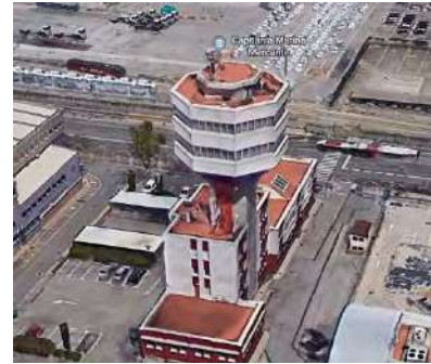
figure 17- Zona Franca Tower
